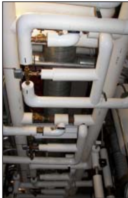
Five Chevy big-block 454s comprise the power plant of the OFA co-generator. One of the engines is shown above. At left is a view, looking up from the floor, of tubing that carries domestic water, boiler water and anti-freeze. In the top photo in the series, OFA head custodian Dan Brink checks the RPM on the outer case of one of the Chevy engines. Each of the 454s run at a steady 1,800-plus RPM.
